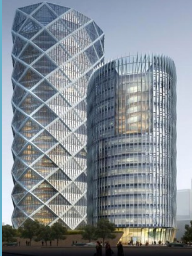
Poly International Plaza, Beijing, China (Skidmore, Owings & Merrill LLP)
